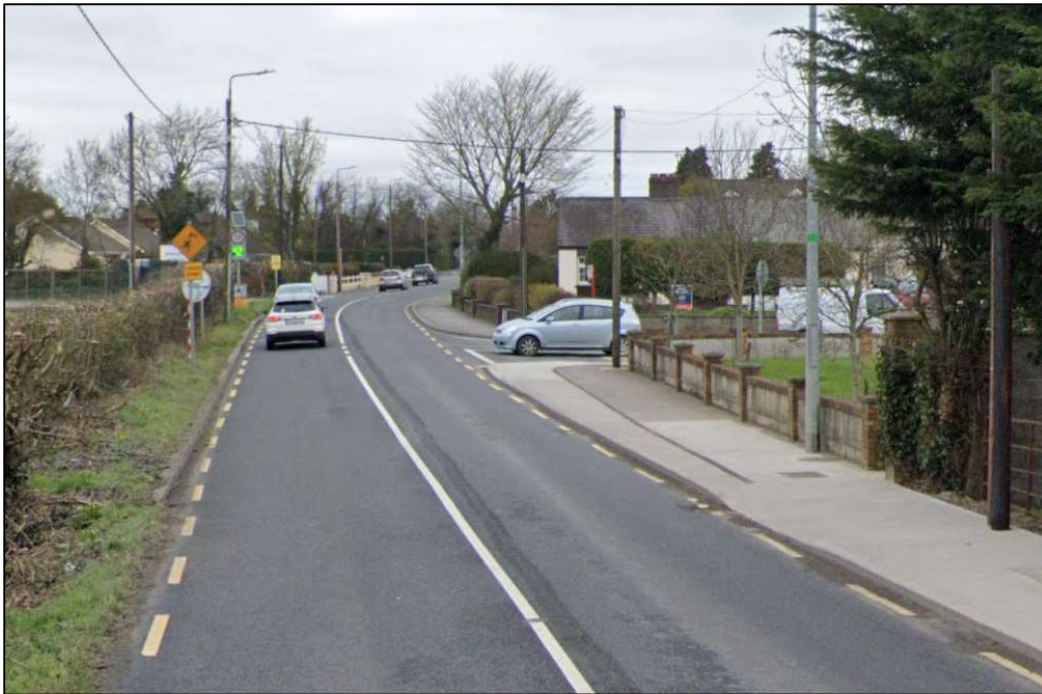
Figure 4: Existing Pedestrian Facilities
